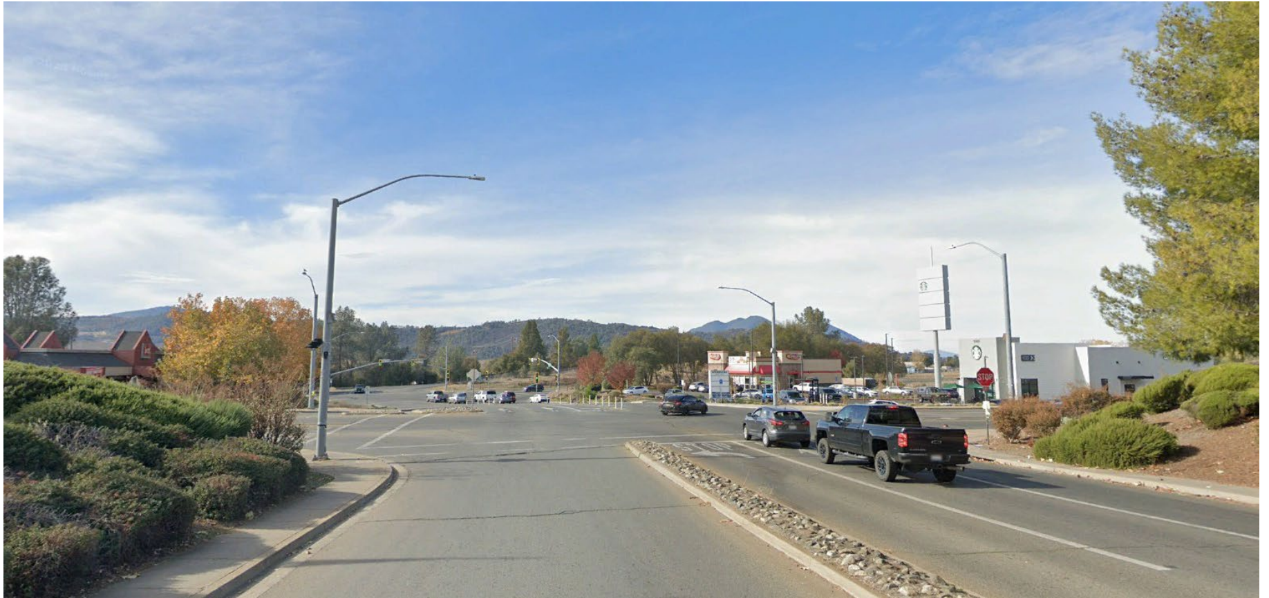
Photo 8: Dam Road Extension Westbound (Looking toward SR 53)
